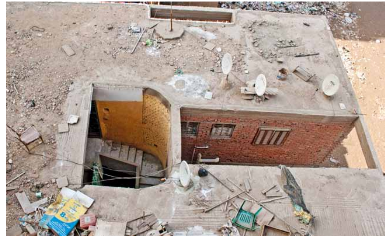
Fig. 03 Building with the two basic types of clearance: a shaft within the building and some slots along two facades
