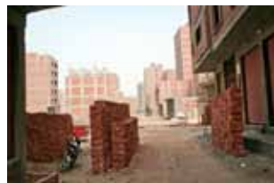
Fig. 01 Construction site, Ard el Lewa (Cairo, 2010)
